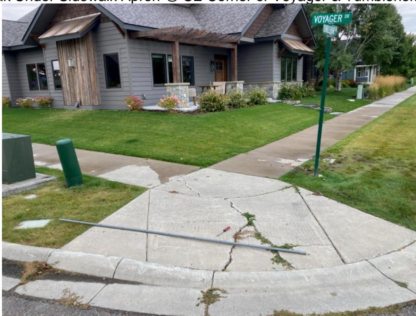
d) Irrigation Leak Under Sidewalk Apron @ SE Corner of Voyager & Tumblehome
